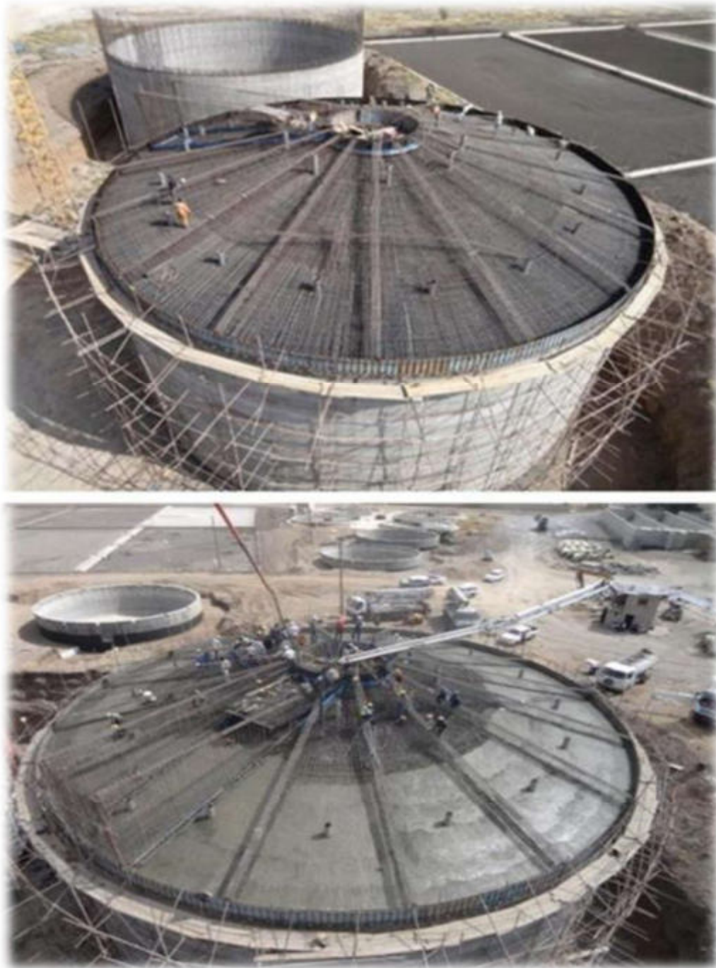
Roof arrangement at Sana'a Yemen
